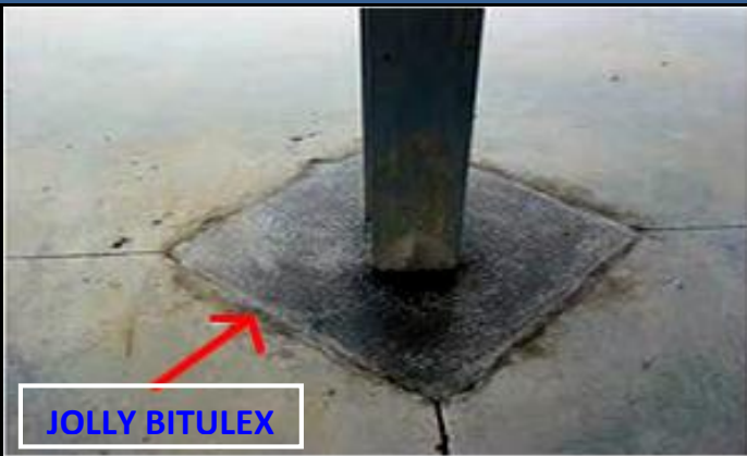
JOLLY EXPANSION JOINT FILLER IN COLUMN JOINTS
