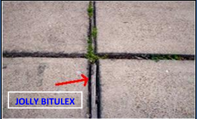
JOLLY EXPANSION JOINT FILLER IN SIDE WALK
